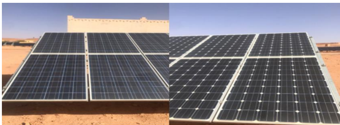
Fig 8. Fixed-Mount Photovoltaic Configuration for Monocrystalline (mc-Si) and Polycrystalline (pc-Si) Subfields.
