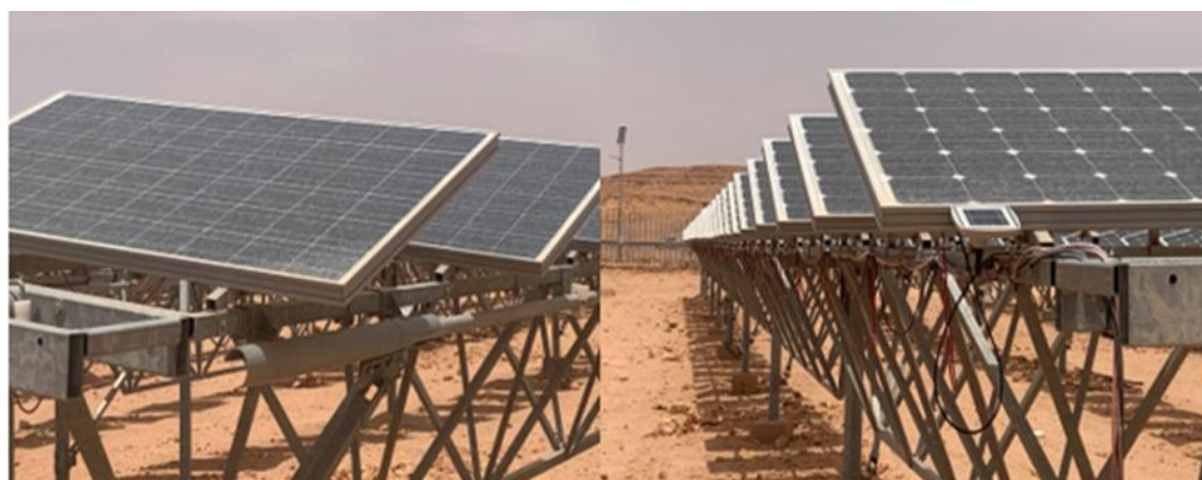
Fig 9. Single-Axis Tracking Structure of the Photovoltaic System in the OUED-NECHOU Subfields for Monocrystalline (mc-Si) and Polycrystalline (pc-Si) Technologies
