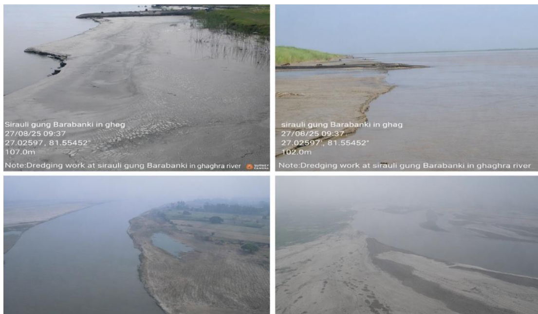
Figure 15. Post Dredging Siltation Near the Bank Protection at Sirauli Goong Barabanki
