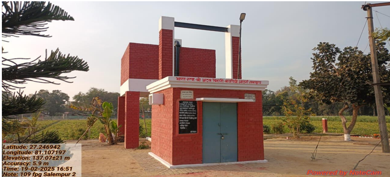
Figure 1: Pilot Installation - Tubewell No. 109 FPG, Village Salempur, Block Fatehpur, Barabanki; Latitude: 27.246942, Longitude: 81.107197)
