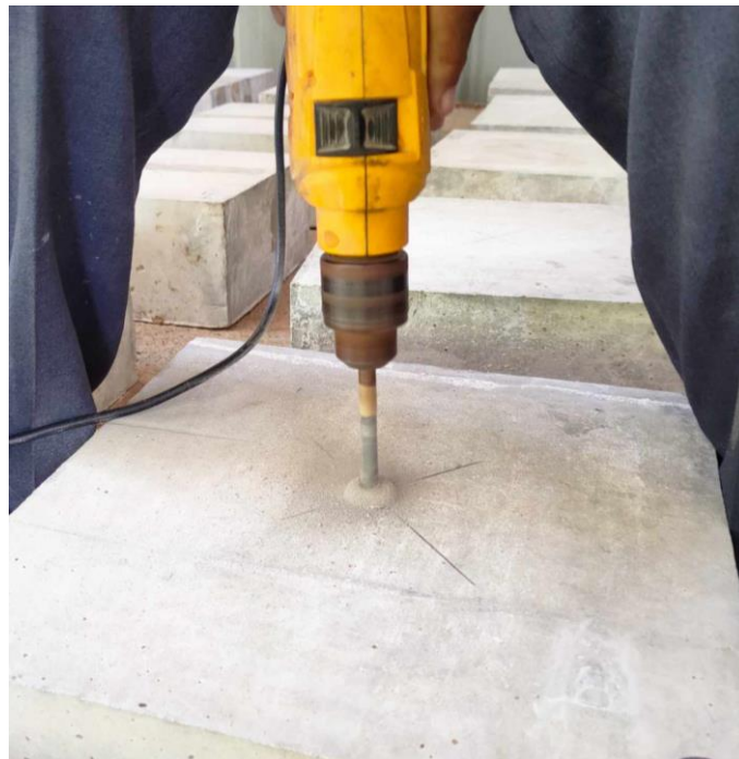
Figure 2 Installation of Expansion Anchor Bolt
