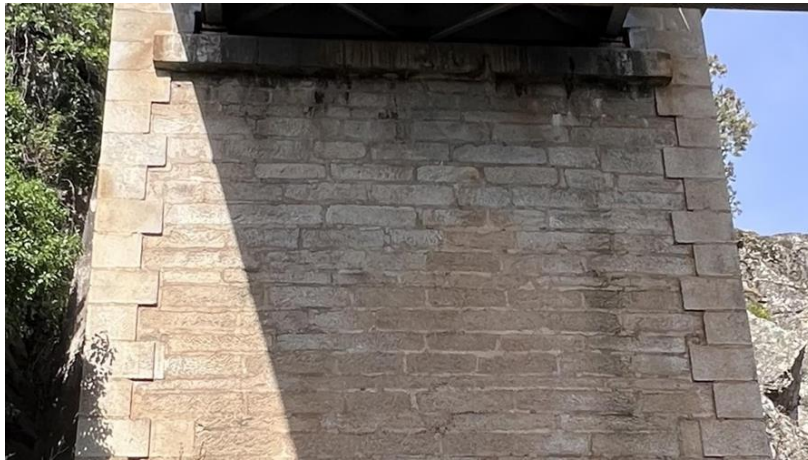
Fig. 12. Face of the second abutment, with traces of runoff water (photograph by the author, taken with a drone).
