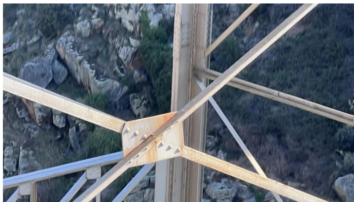
Fig. 16. Corrosion located in one of the braces of the palisade at the west end of the Bridge, upstream side (photograph by the author, taken with drone).
