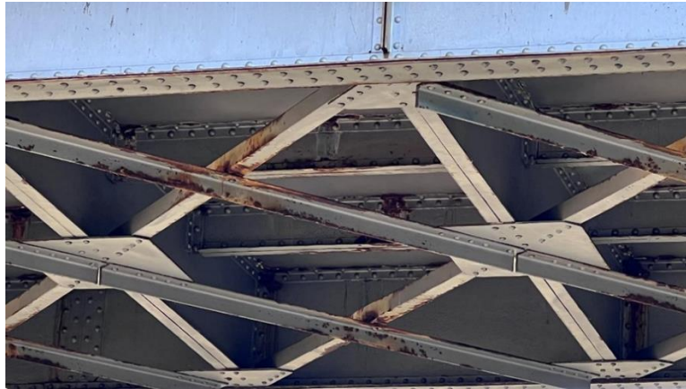
Fig. 22. Detailed view of a section of the deck, where localized corrosion of several elements can be observed (photograph by the author, taken with a drone).
