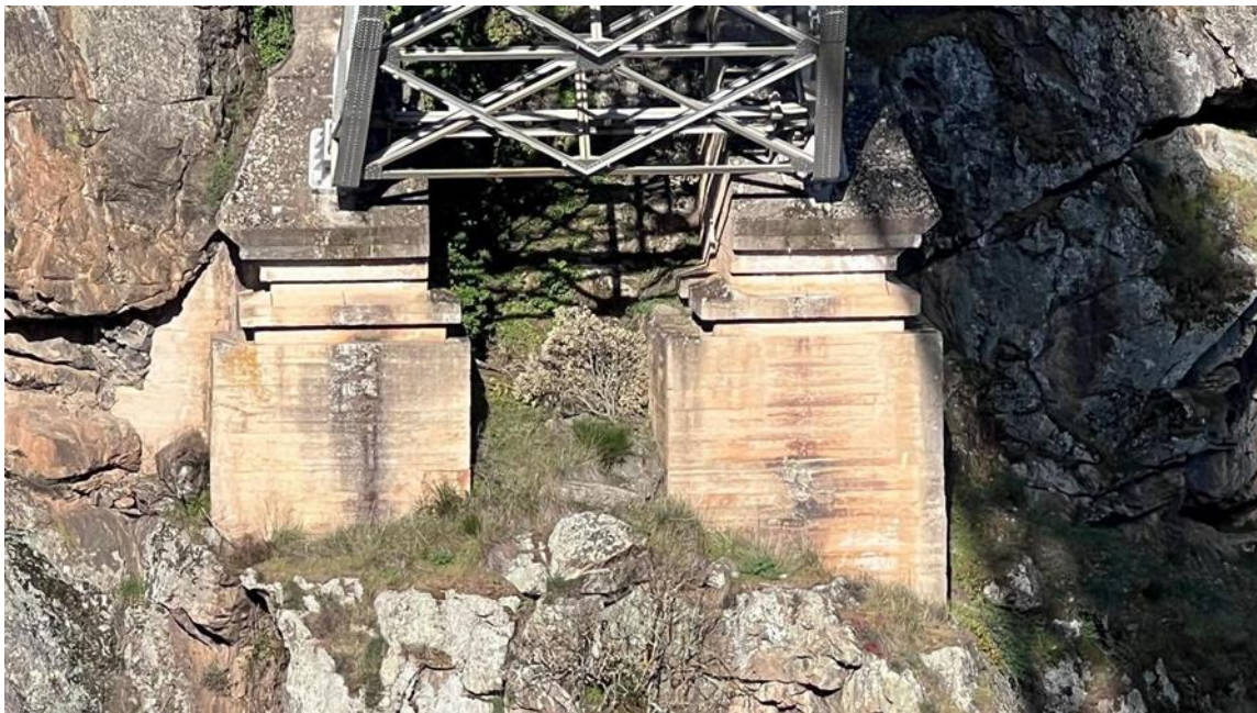
Fig. 8. Arch supports on direct concrete foundations in the area of the second abutment (photograph by the author, taken with a drone).
