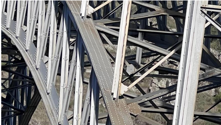
Fig. 9. Examples of upright supports on the arch, through platforms anchored with bolts, on the upstream side (photograph by the author, taken with drone).
