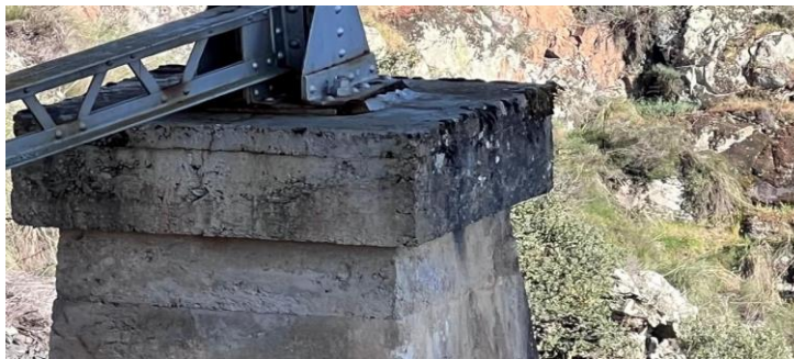
Fig. 15. Loss of one of the anchor heads in palisade 7, downstream side (photograph by author, taken with drone).
