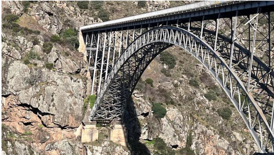
Fig. 7. Partial view of the Bridge, from the south side (upstream side), where you can see the constitutive arch and, in the background, the second abutment, with its corresponding support palisades (photograph by the author, taken with a drone).
