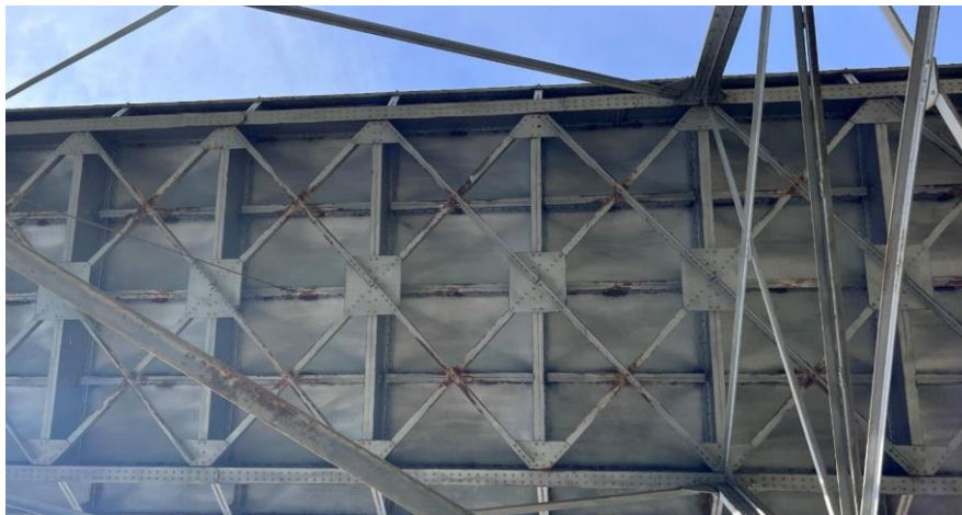
Fig. 21. View from the underside of a section of the deck, where a multitude of elements with symptoms of localized corrosion can be seen (photograph by the author, taken with a drone).
