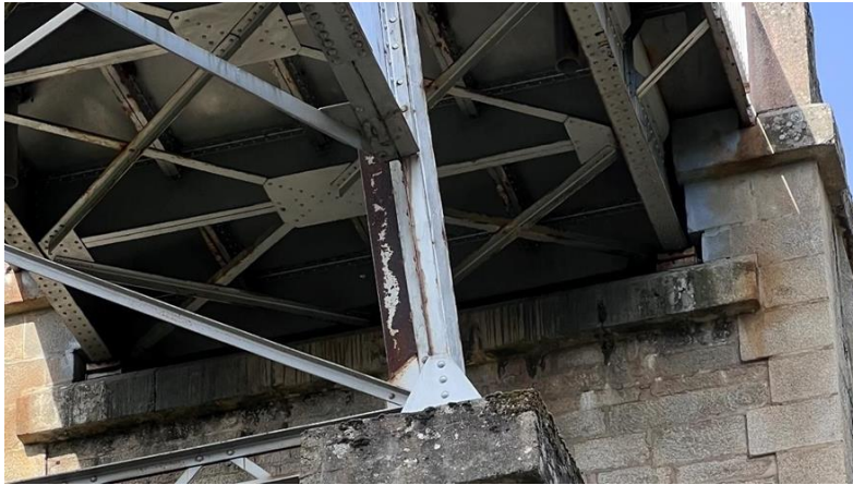
Fig. 14. Corrosion in palisade number 7, the closest to the second abutment, downstream side (photograph by the author, taken with a drone).
