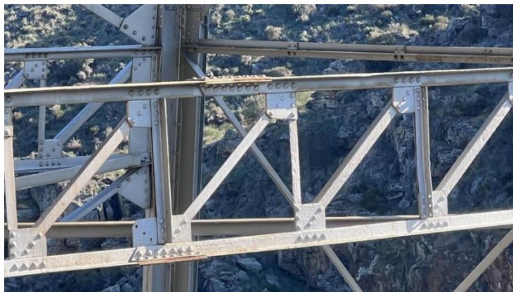
Fig. 19. Detail of a section of the arch, with spot corrosion located in the joint areas (photograph by the author, taken with a drone).
