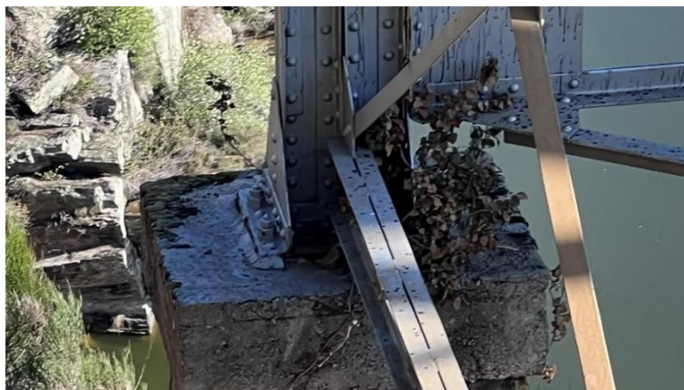
Fig. 13. Presence of organic matter and vegetation in the concrete support die of palisade 6, downstream side (photograph by the author, taken with a drone).
