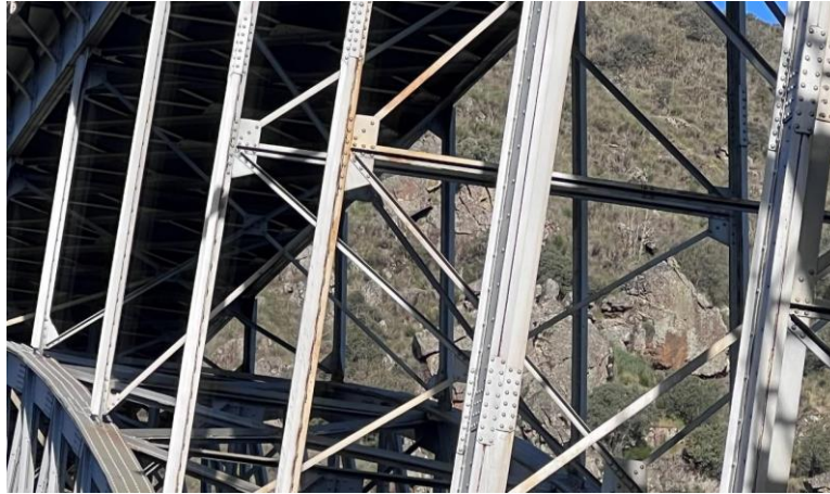
Fig. 20. Detail of corrosion in one of the uprights above the arch (photograph by the author, taken with a drone).
