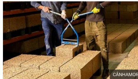
Fig.5 Hemp bricks are made from hemp fiber, limestone powder and water.
