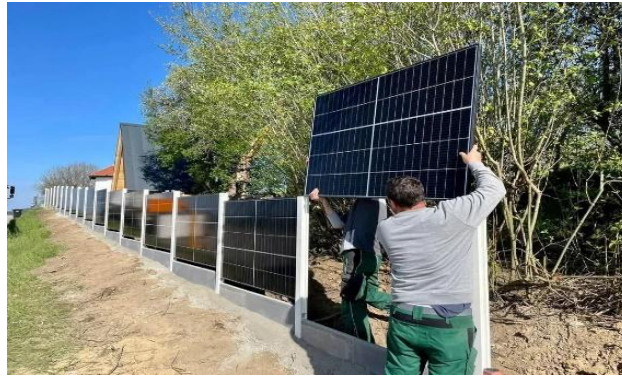
Fig.7 using solar panels to build a wall to save energy and building materials.
