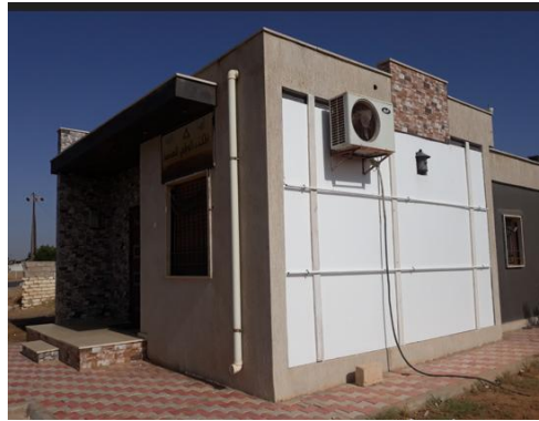
Figure 10: Building Facade with External Thermal Insulation Panels Installed
