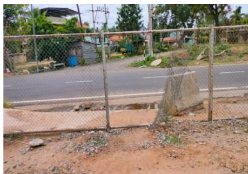
Fig 1. Broken barricade from hit of the heavy vehicle
