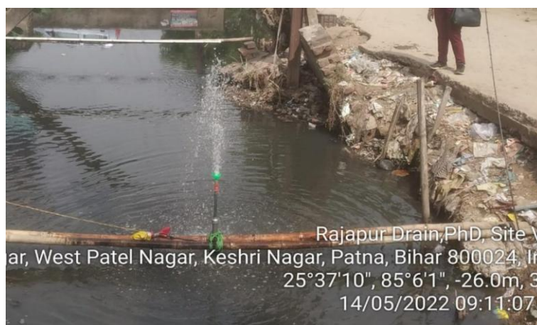
Figure 2: Reaeration and biological product dosing at initial point of Rajapur drain
