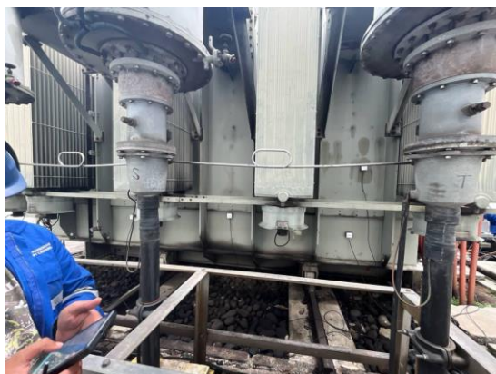
Figure 10. Installation of 4 AE Sensors
